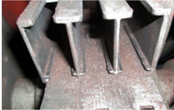
Cleaning of power slip ring unit
