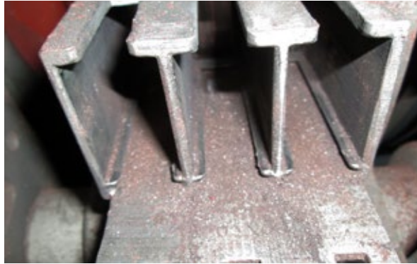
Cleaning of power slip ring unit
